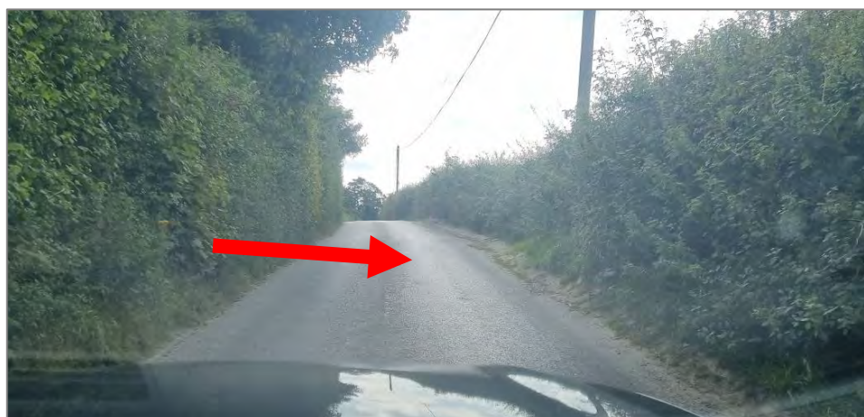
Figure 2-9: Verge Over-Run
